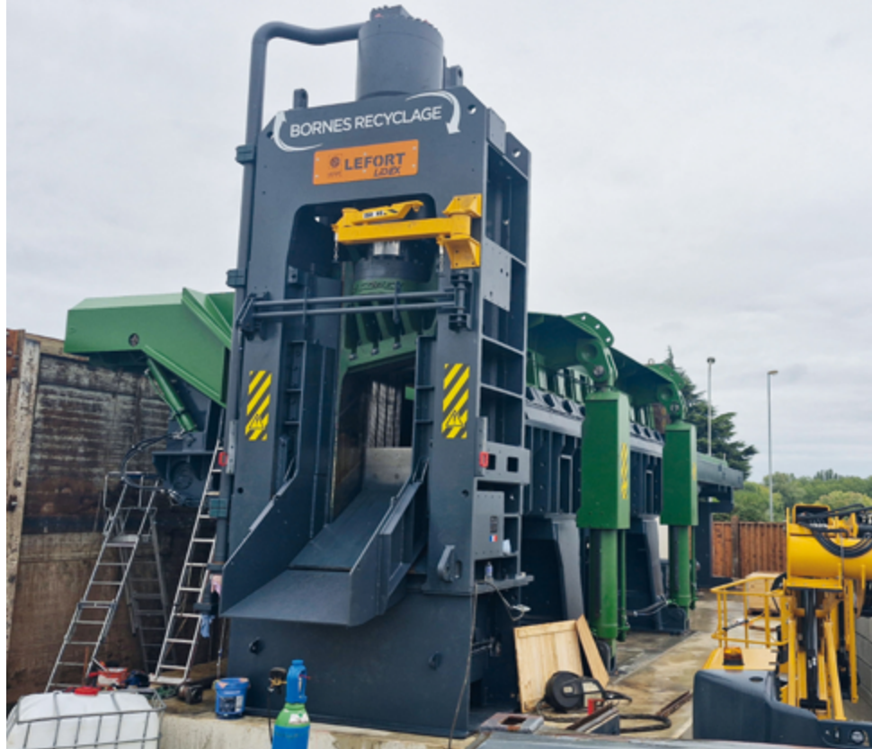
End of the on-site assembly of the LIDEX
